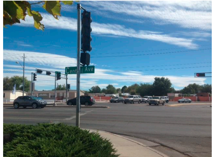
Figure 5. Lack of a marked sidewalk at CZ intersection.
