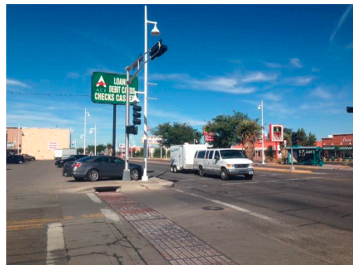
Figure 3. Lack of curb cuts and faded crosswalk in SM3.
