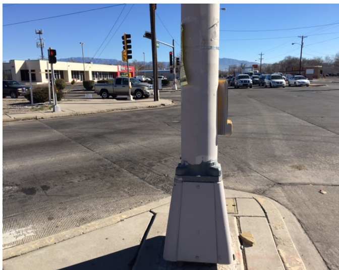
Figure 15. Difficult-to-reach buttons, faded crosswalks, and a non-working signal lowered scores for all segments connected to the Five Points Road intersection (B1–B6 and B9 & 10).
