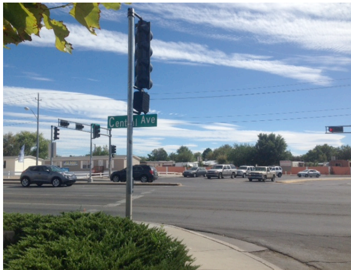
Figure 10. Photograph illustrating the lack of a marked crosswalk on the East side of the intersection at Central Ave and Zuni Rd.
