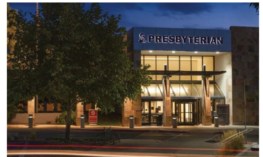
Presbyterian Kaseman Hospital in Albuquerque, NM
