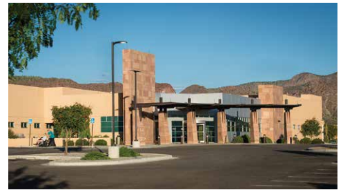
Socorro General Hospital in Socorro, NM
